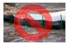
Installing silt fence in a direct flow is wrong for two basic reasons, either the fence will fail immediately, rendering it ineffective, or the water will pile up behind it and fail catastrophically, taking out everything downstream...
